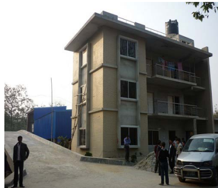
Latex Processing Factory
